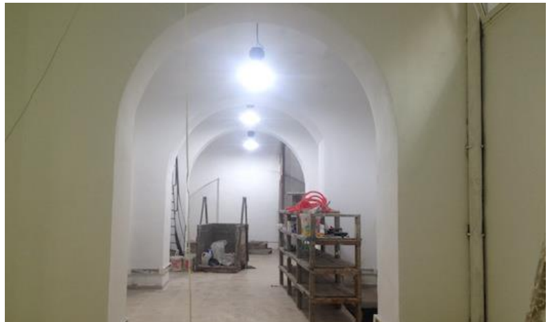
Renovations at the Office of Sylabs
